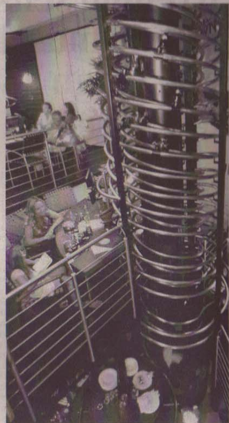
An ingenious system of spiralling rails brings the food from the kitchen in the room above to the diners
